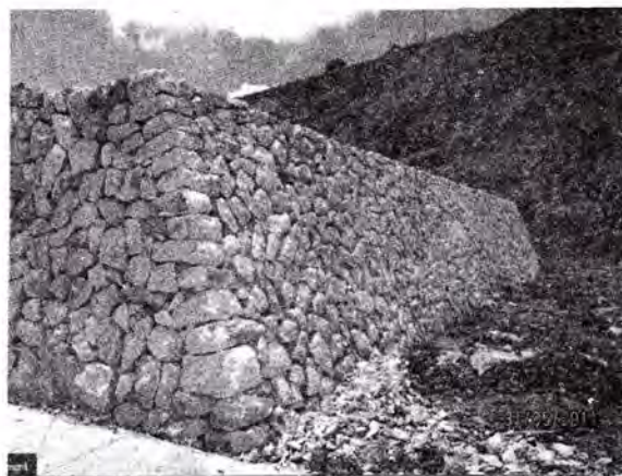
The retaining wall/slope protection for the water cistem.
